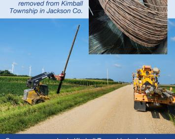
Crews remove poles in Kimball Township in Jackson County. Overhead line was replaced with new underground. Some of the line and poles in the area were original construction.
